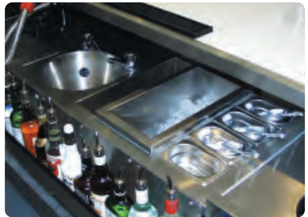
Typical bar with insulated ice well, condiment pots, hand wash sink and speed rail.
