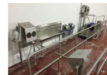
Typical Hygiene Entrance Arrangement
